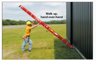
First check for sufficient overhead clearance and make sure there are no power lines. Carefully erect the ladder by "walking" it up to a vertical position. Be sure the bottom is securely blocked against a fixed object or "footed" by another person.
