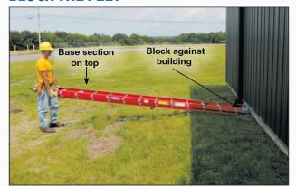
The ladder should be closed. Position the ladder with the base section on top of the fly section. Block or "foot" the ladder against the base of the building or another secure object.
