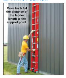
Move the ladder away from the building so that it can be set at the proper angle. Carefully and firmly grip the ladder before moving - keep it vertical.
