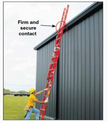
Carefully lean ladder against building at the correct 75-1/2° angle. The base should be 1 foot out for each 4 feet of ladder length to the upper support point. Extend the ladder 3 feet above the roof edge for access. Be sure both end caps or
