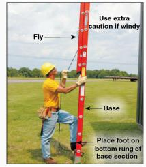
Carefully raise the fly section using the rope and pulley system. After the bottom rung of the fly section clears the bottom rung of the base section, place one foot on the base rung to provide continuous firm footing.
