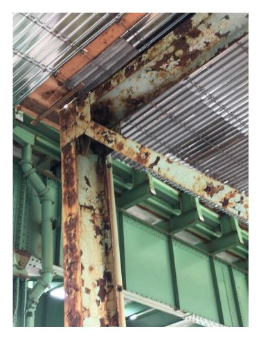
The Chelsea Viaduct is considered to be in even worse condition. Large portions of the structural steel support are rusted out and pose immediate concerns. When complete, these efforts will remove 15% of the structurally deficient bridge deck in the Commonwealth of Massachusetts.
