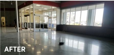
Each floor section was ready for foot traffic in two to three hours and for grinding in 24 hours. During grinding and polishing, the crew started with a 30/40 metal soft bond diamond grit and worked their way up to a 1,500-grit polish for a high-gloss finish. The final steps included applying a guard and burnishing.
