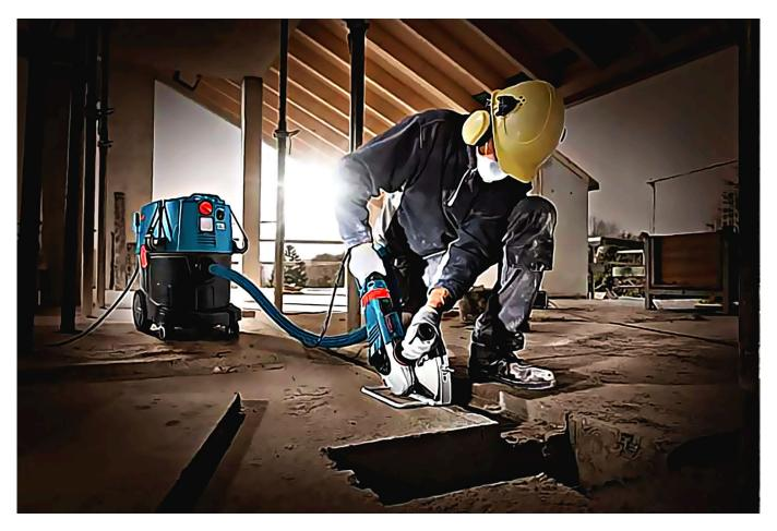
Fortunately, contractors have discovered that worker exposure to silica can be drastically reduced by using the new generation of power tools with a dust attachment/accessory and dust extractors.
