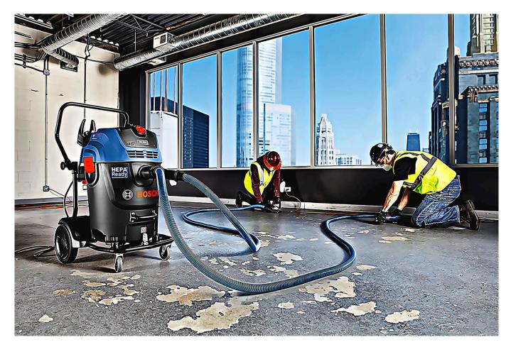
There's an additional benefit with the larger extraction capacity. The OSHA standards do not specify that only one grinder must be dedicated to a single dust extractor. This means workers can legally use a <u>Y-Connector</u> that allows the use of two grinders on one 300CFM dust extractor. Talk about productive!
