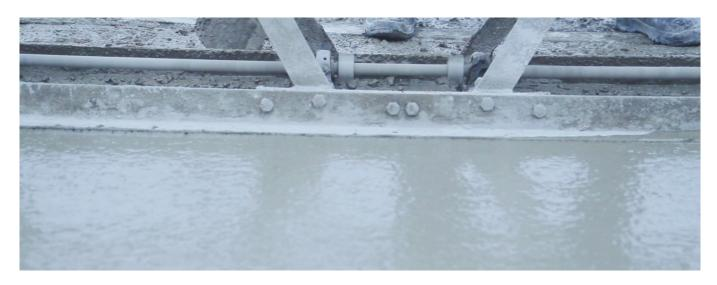
Consolidation of concrete through internal vibration guarantees greater density and strength of the concrete. It also improves the bond with the incorporated reinforcement steel and construction joints. With less honeycombing, the concrete will have a longer life and greater durability. All of these advantages of concrete consolidation can save contractors significant time and money after the pour.
