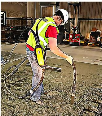
concrete at the optimal time and in a systematic manner. The vibrator should be submerged into wet concrete as the slump is moving into place or just after it levels out a bit. The operator places the vibrator into the concrete and allows it to sink under its own weight; it is recommended to leave the vibrator in for up to 15 seconds before being withdrawn slowly. As it is withdrawn, the air bubbles will rise to the surface around the vibrator's head.
