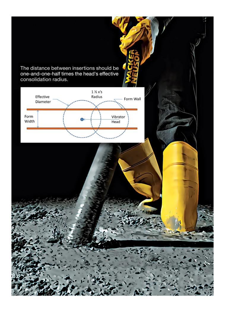
The vibrator itself must be in consistent, continual motion by the operator in order to reach all the potential air pockets. Operating an internal vibrator takes some training. An effective operator can visually tell when the air bubbles cease to come to the surface and when the thin film of water rises.
